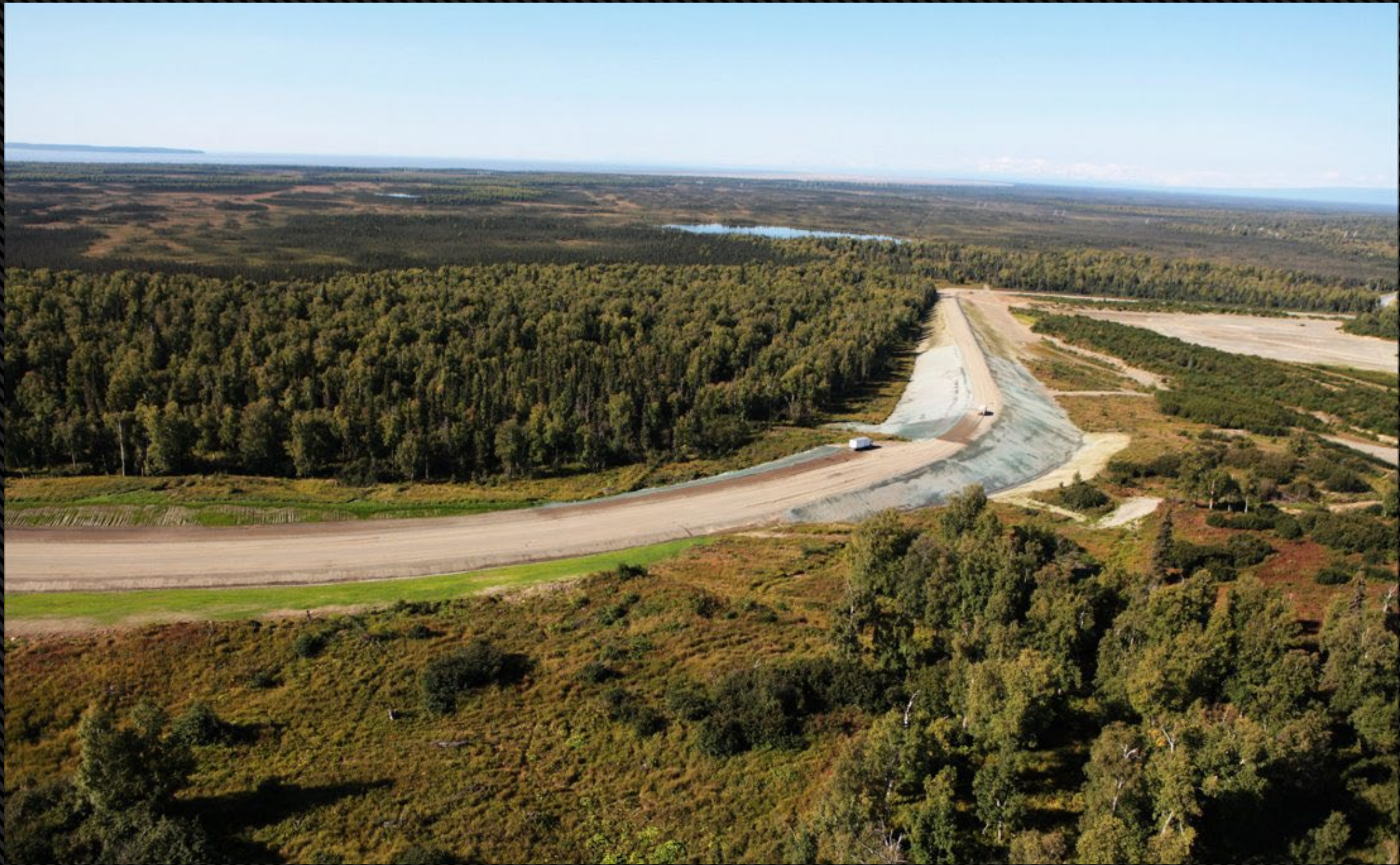
Port Mac Railbed
