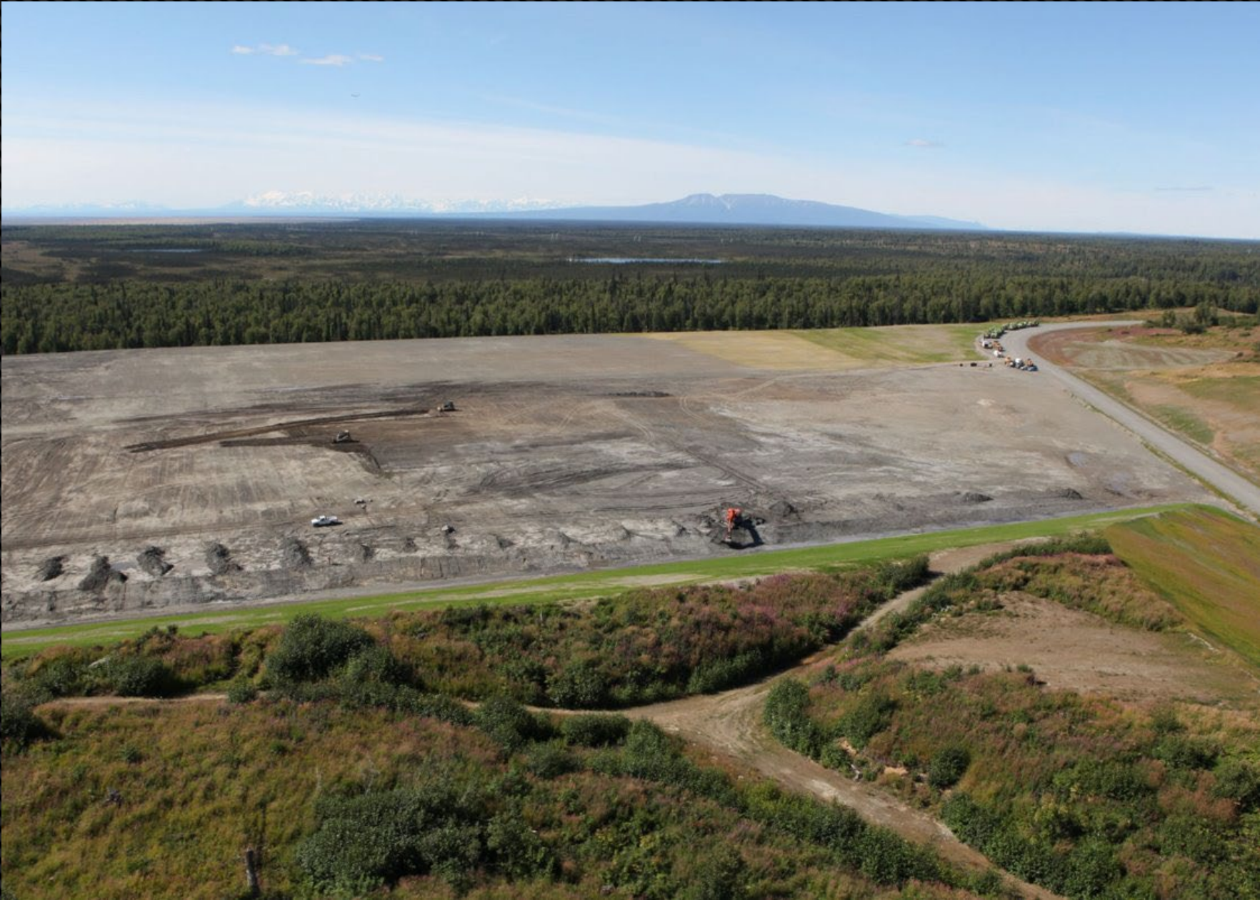
Port Mac - Storage Area
