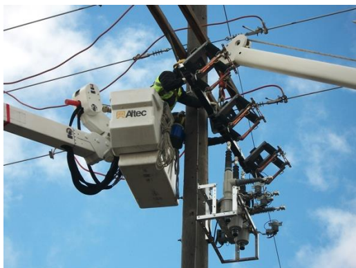
Lay the foundation for a regional Smart Grid
