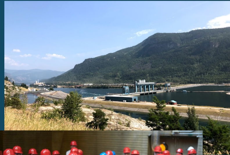
Hugh Keenleyside Dam in British Columbia
