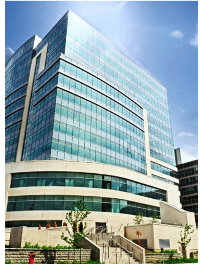
Place Victoria, Gatineau, built with Contempra-based concrete
